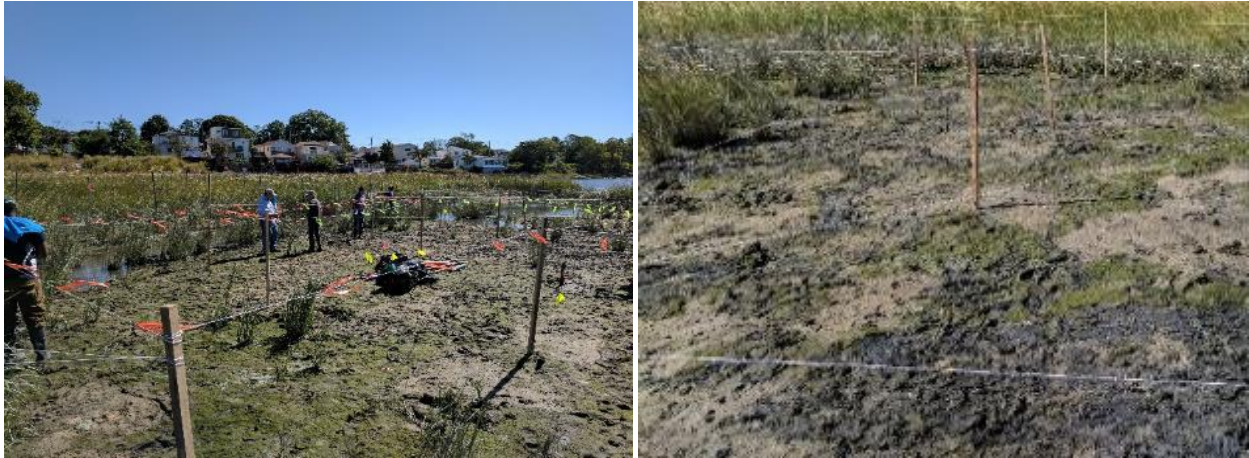
Figure 21. Example photos of algae colonization (left) and goose fence installation at Soundview Park in the Bronx where plants were lost due to goose herbivory several years following restoration. Stakes with nylon string and attached bright flagging installed by volunteers (left). Algae on the marsh surface (right).
