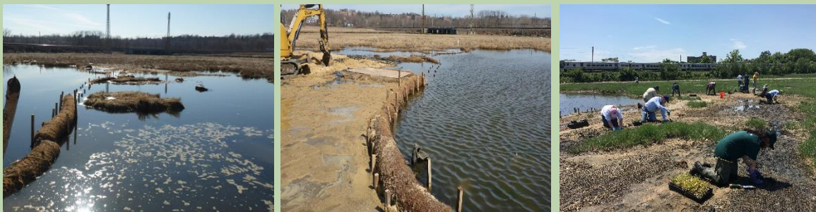
Figure 17. Salt marsh restoration at Alley Creek in Queens, NY, through placement of clean sediment where open water persists. Setting coir log along the flooded former marsh early April 2017 (left). Placing and marsh mats to access the marsh with machinery mid- April 2017 (middle). Planting Spartina alterniflora with staff and volunteers, June 2017 (right).
