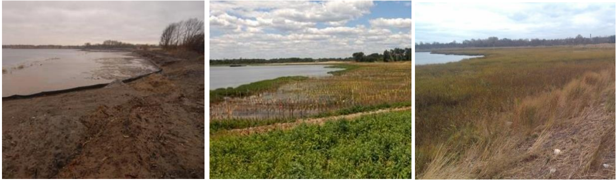
Figure 14. Gerritsen Creek restoration during excavation ca. 2010 (left), immediately after planting ca. 2011 (middle), and immediately after Hurricane Sandy ca. 2012 (right). Clean soil existed under excavated fill, so no clean sand was placed.
