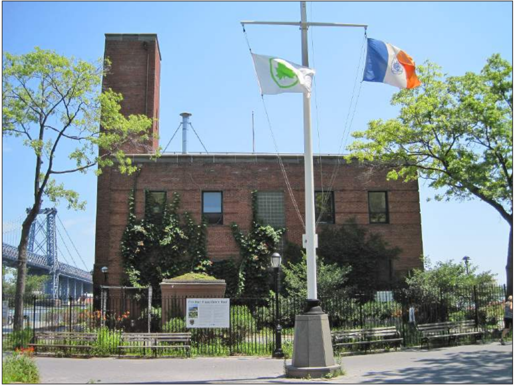
Fireboat house (#4). View within East River Park 5
