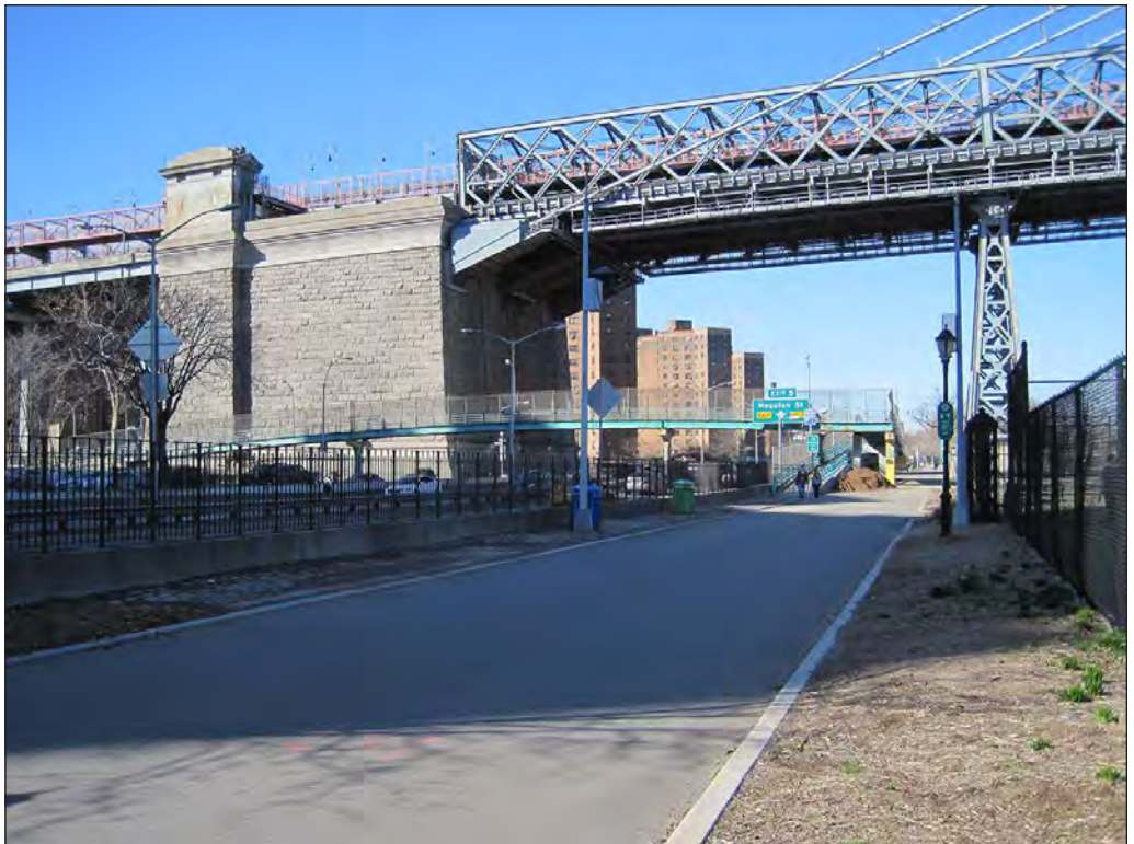
Delancey Street pedestrian bridge, view north 4
