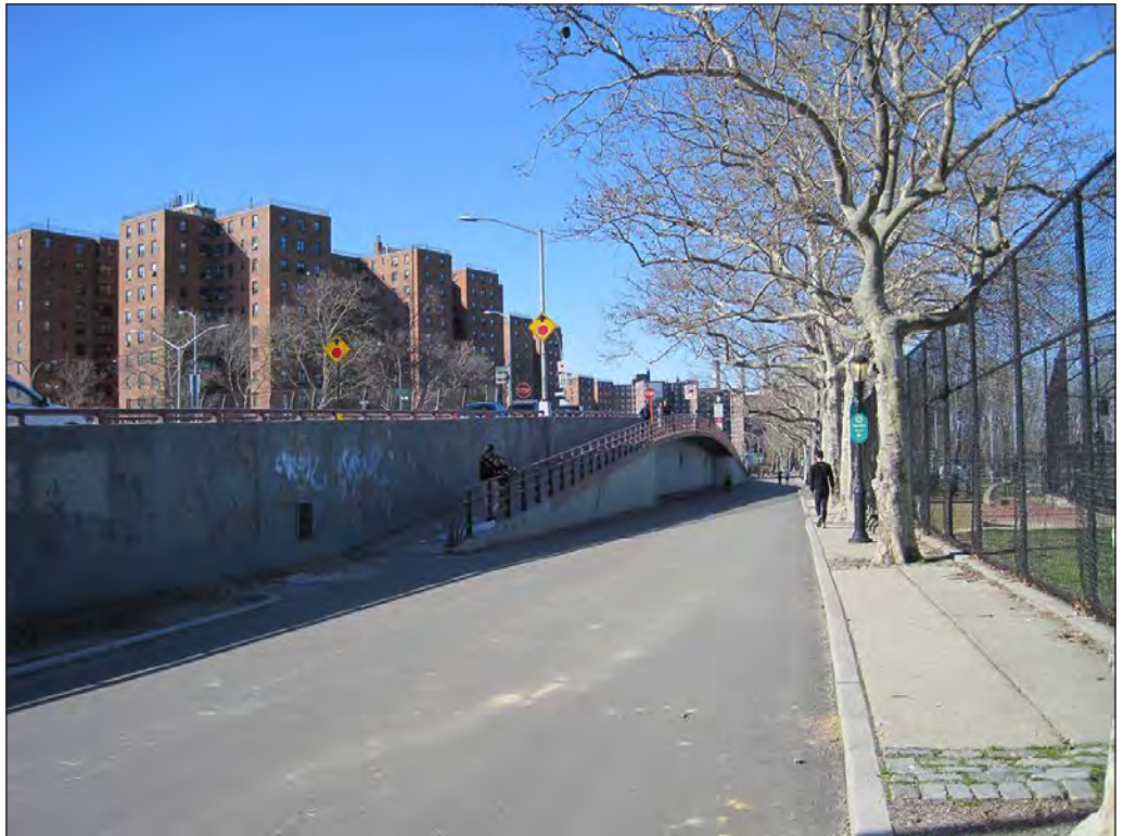
East Houston Street overpass, view north 5
