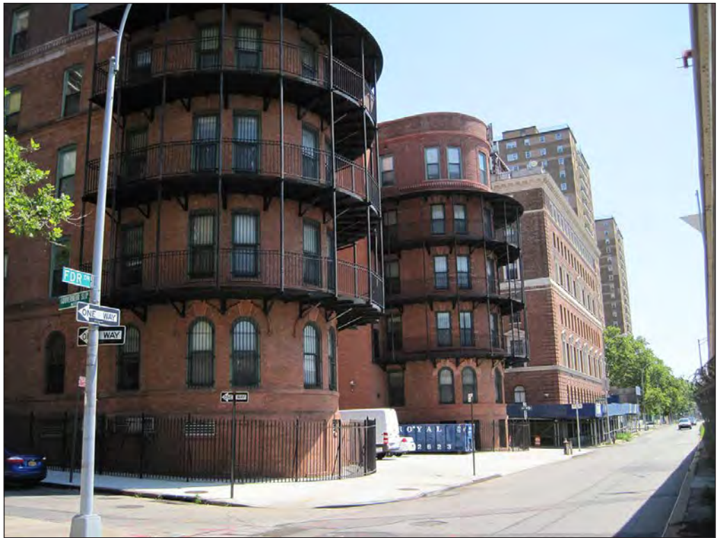
View east on South Street from Gouverneur Slip East 65
