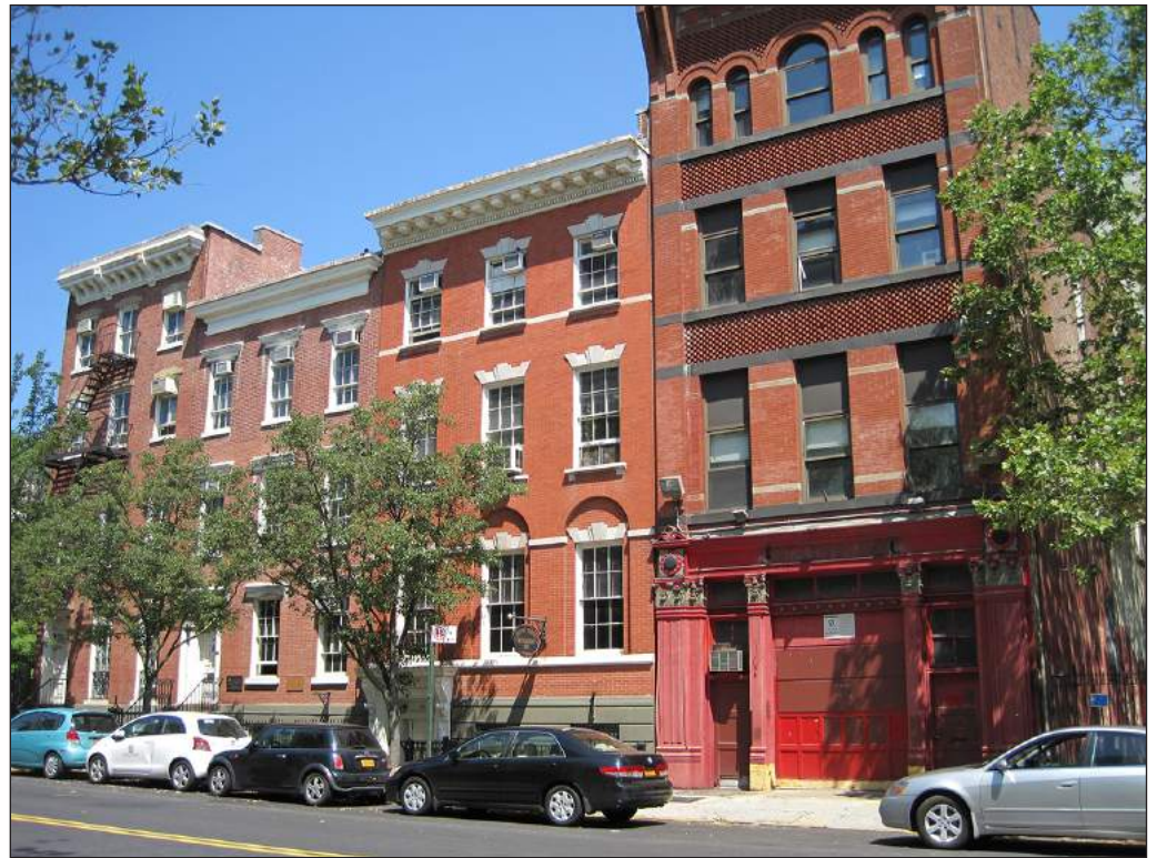
Henry Street Settlement, 263-267 Henry Street (#8) 13
