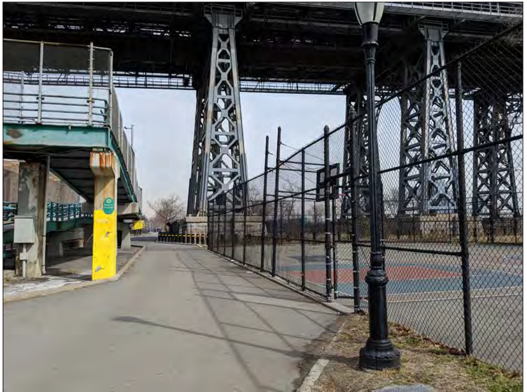
Basketball court at Delancey Street, view north 21
