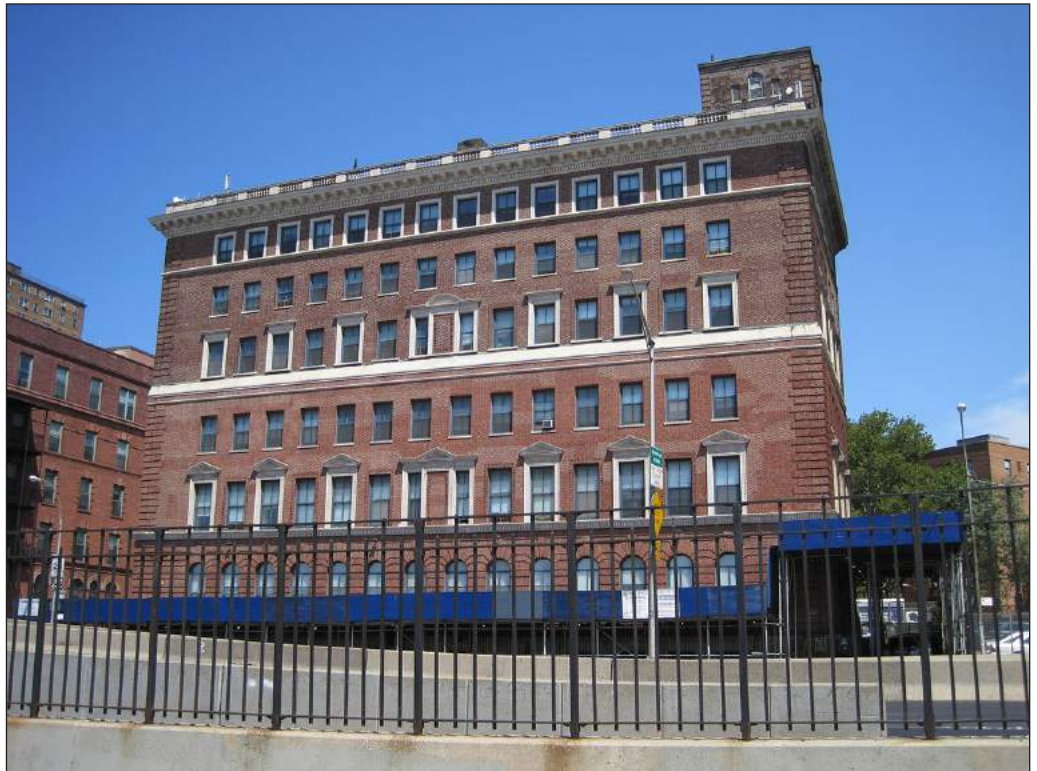
Gouverneur Hospital Dispensary (#6). Water Street façade 10
