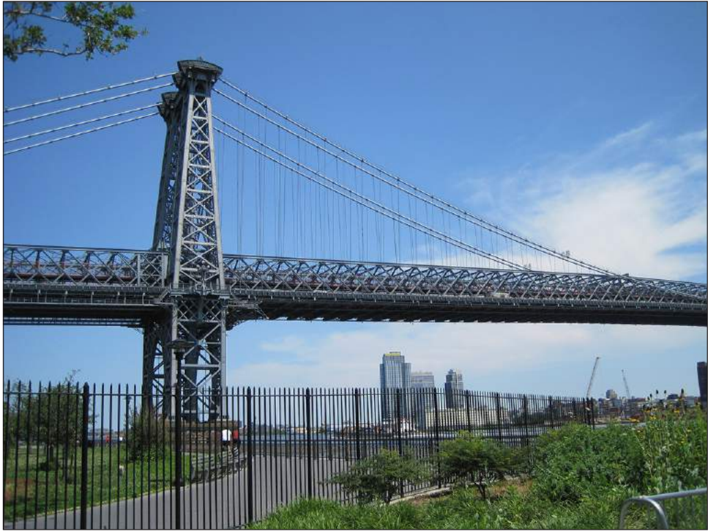
Williamsburg Bridge (#2). View north within East River Park 3
