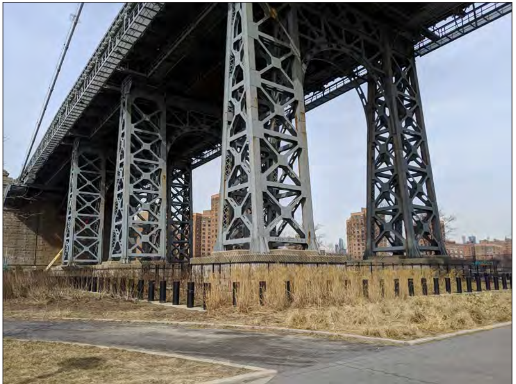
Williamsburg Bridge footings, view northwest from esplanade 22
