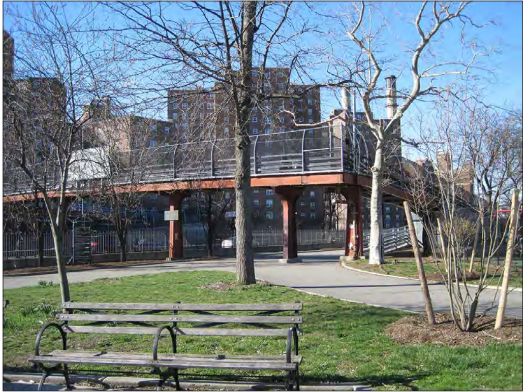
East 10th Street pedestrian bridge, view north 7
