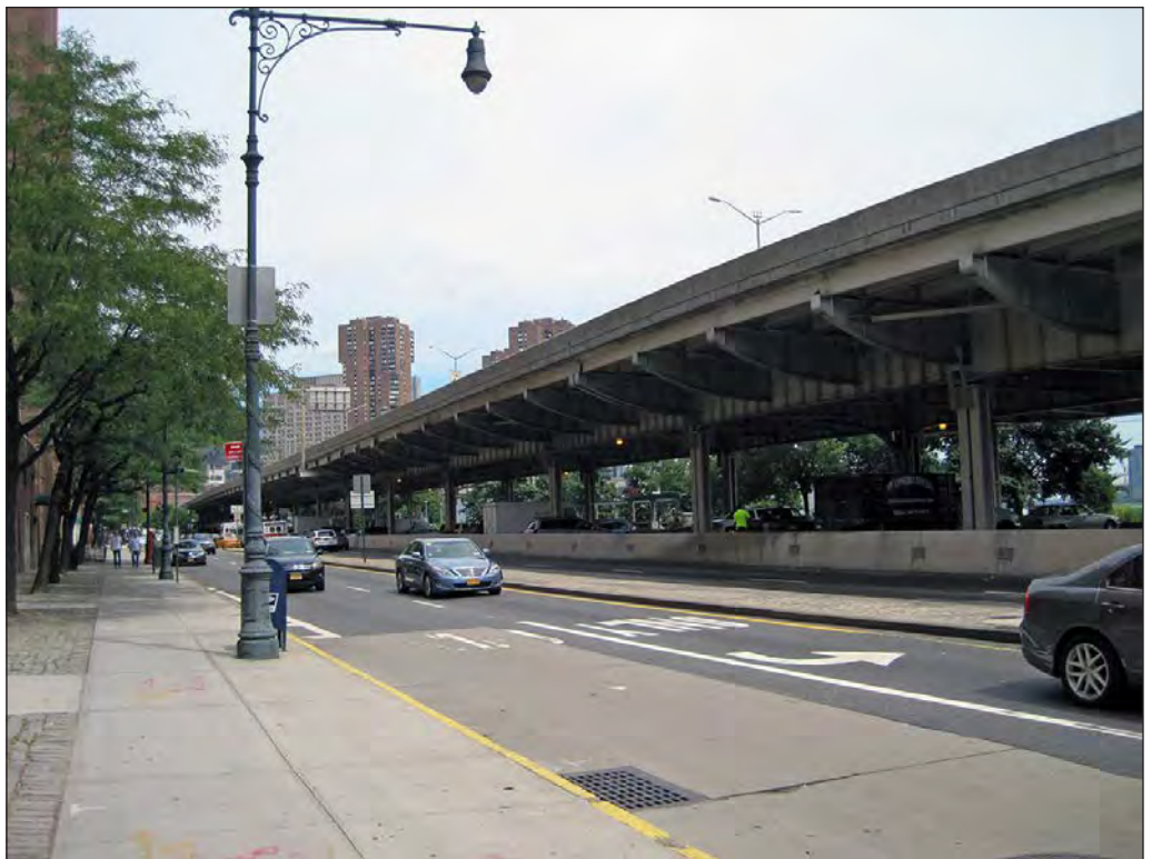
FDR Drive, view north at Avenue C 45
