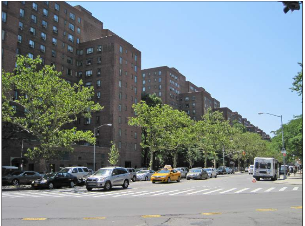
Stuyvesant Town (#16). View southwest on West 20th Street 22
