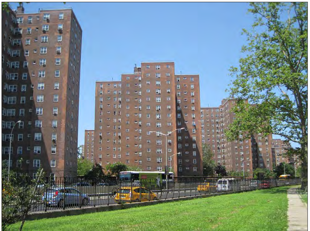
Jacob Riis Houses, view northwest from East River Park 73
