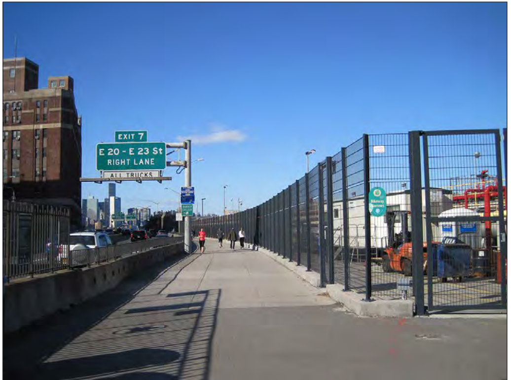
Walkway adjacent to Con Ed facility, view north 44
