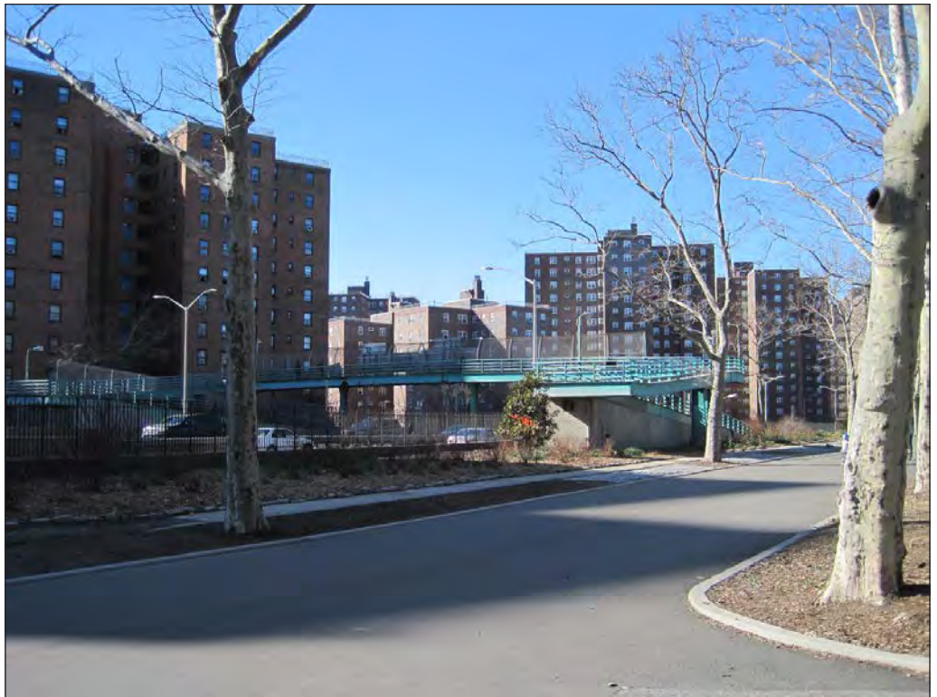
East 6th Street pedestrian bridge, view north 6
