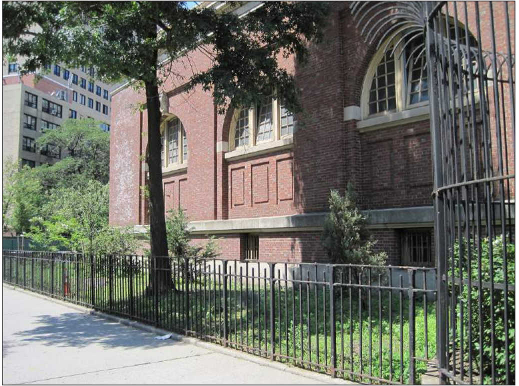
Asser Levy Public Baths (#12). South (West 23rd Street) façade 18
