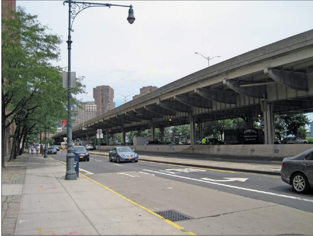
FDR Drive (#1). View north at Avenue C 7
