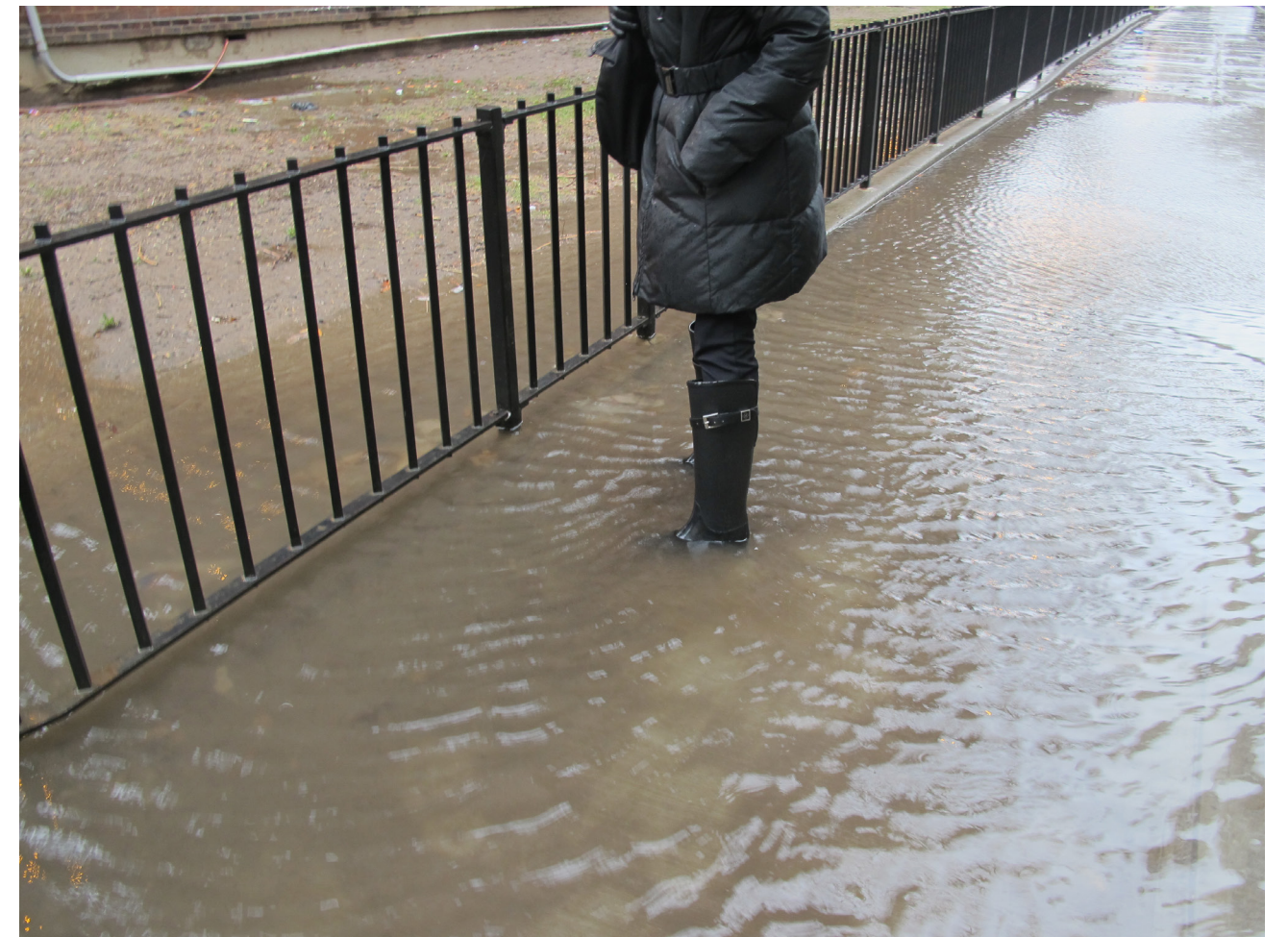
Inland ponding on East 103rd Street after a storm in March 2018.
