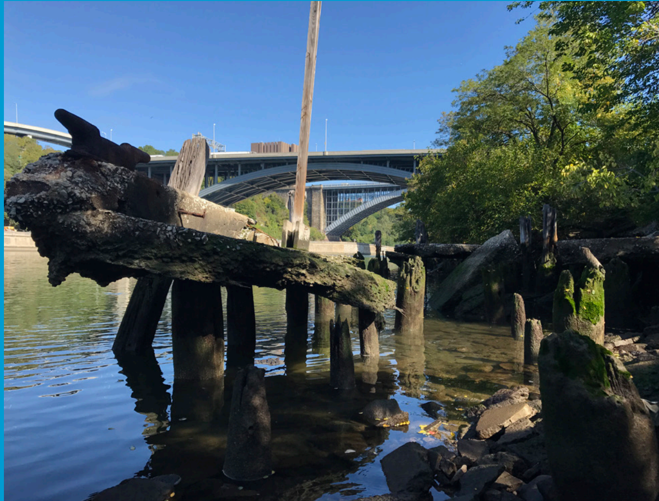
Remnant pier structures along the shoreline at Bridge Park South, 2017.
