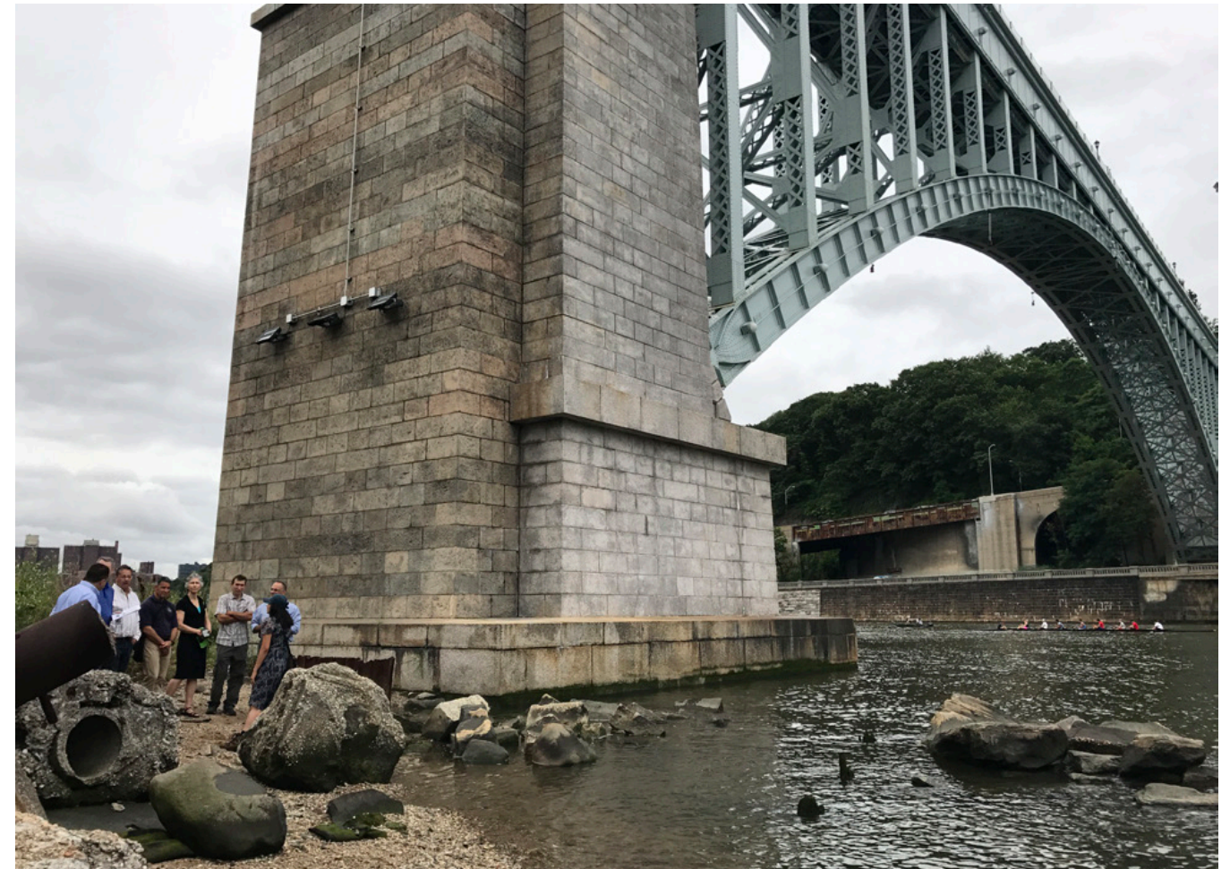
Discussing Harlem River shoreline restoration opportunities at the base of the High Bridge.
