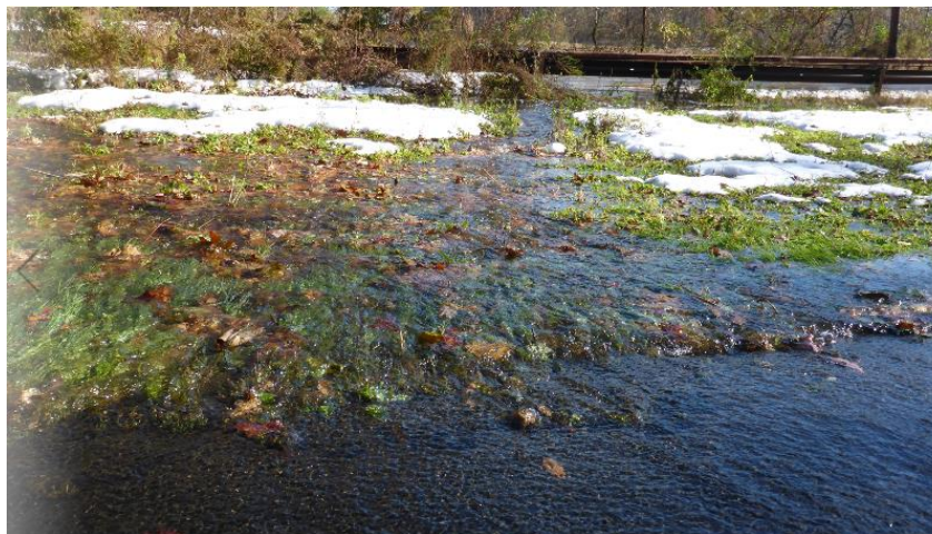
d) Undersized culvert causing flooding at Shore Road in the Bronx.
