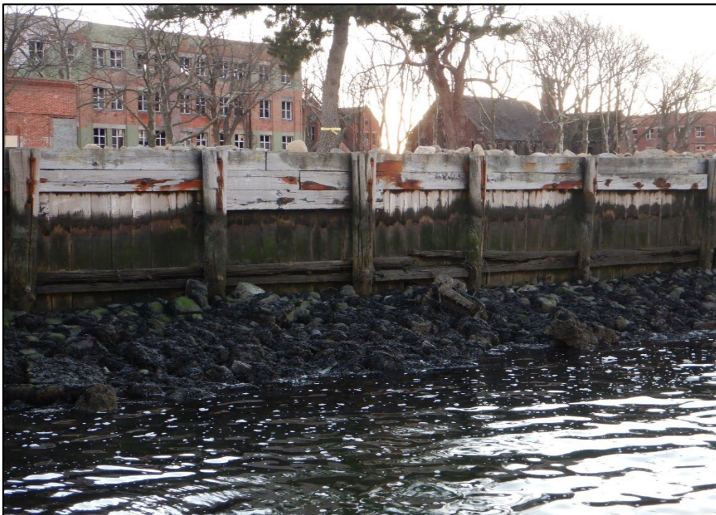
Photo 2-4. Typical view of the Hart Island Ferry Dock Shoreline, looking east.
