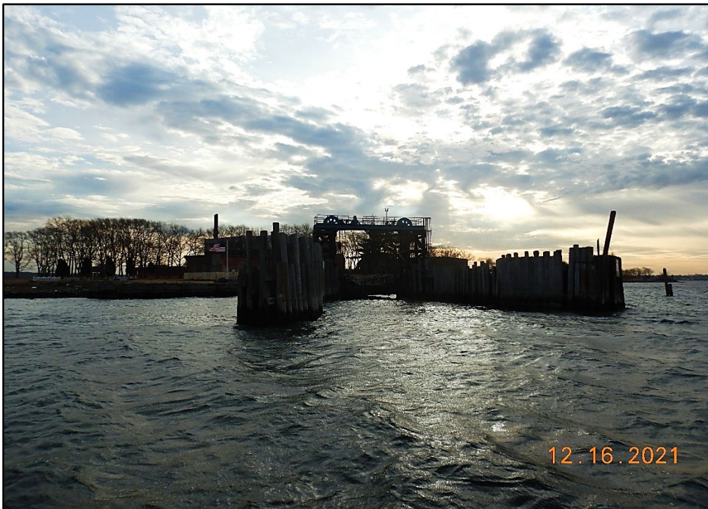
Photo 2-8. General view of the Hart Island Ferry Dock, looking east.
