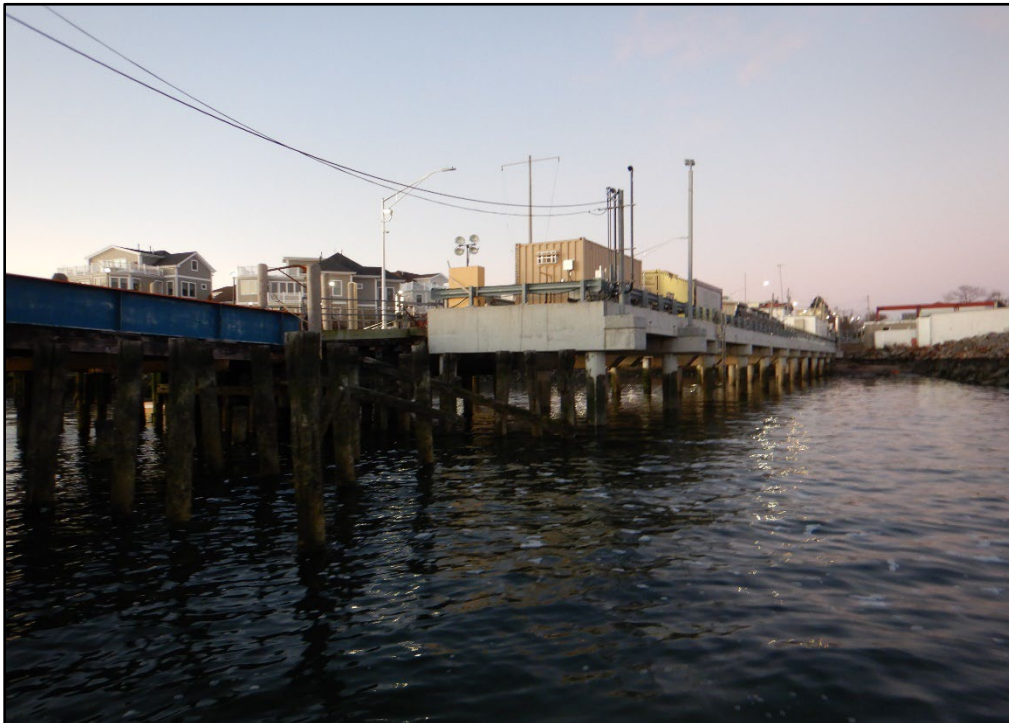
Photo 2-6. General view of the Fordham Street Pier at City Island, looking west.
