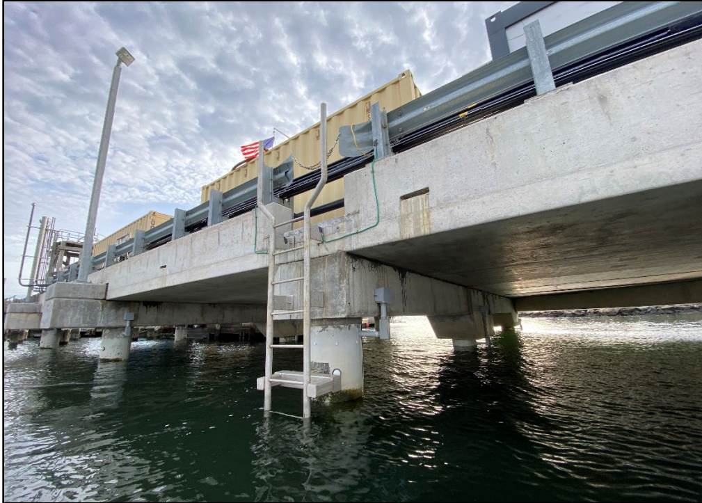
Photo 3.2-1. Newly constructed Fordham Street Pier with epoxy encased piles, concrete pile caps, a concrete deck with steel safety ladders, street lights, and a safety guard rail, looking southeast.
