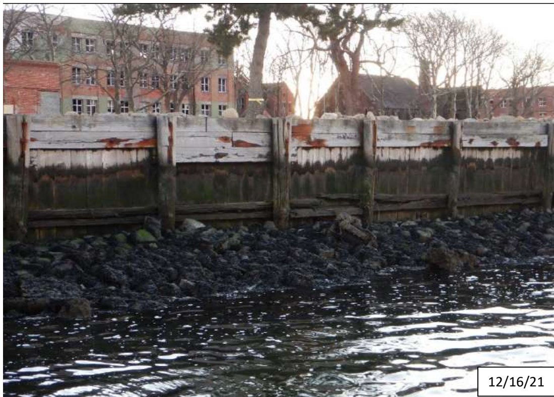
Figure 28 – Photo of Bulkhead at Hart Island Ferry Dock Shoreline
