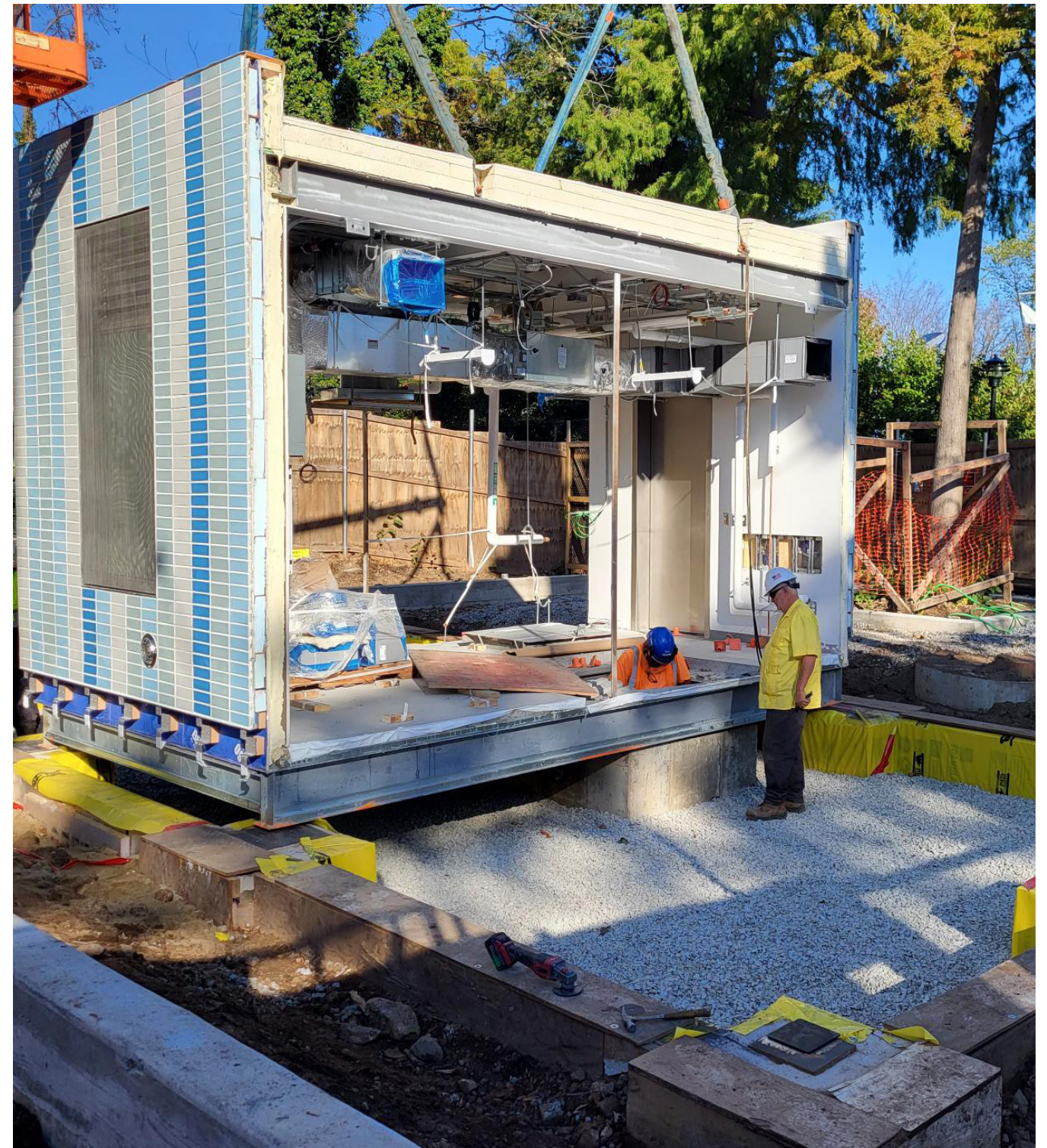
Luis R. Lopez Playground, Modular Public Restroom Building, Staten Island
