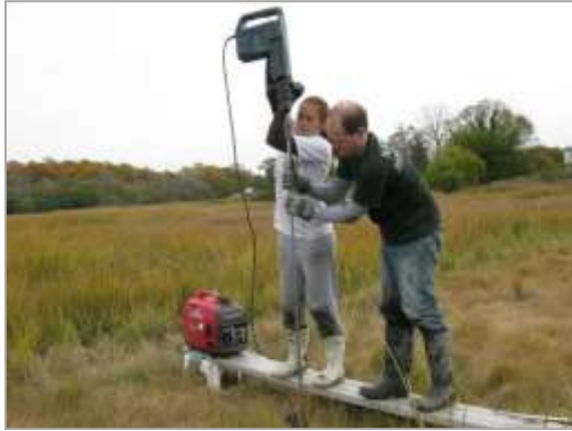
Figure 2. Installation of steel rods (4 foot sections are repeatedly threaded into the ground until point of refusal). A receiver is added the top and stabilized with concrete.
