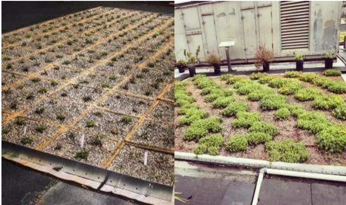
BIOtray System Initial Installation (left) and After BIOtray Break Down (right)
