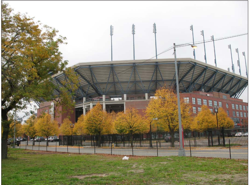
Existing/no action conditions
