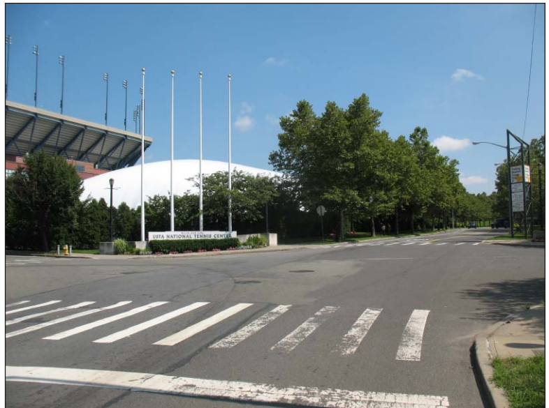
Parking Lot A, view south from Meridian Road 3
