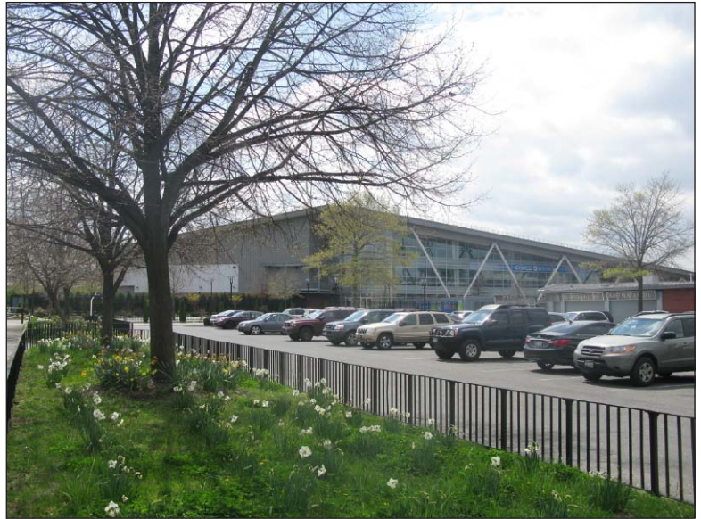
Indoor Tennis Center and Lot B, view south from Meridian Road 1
