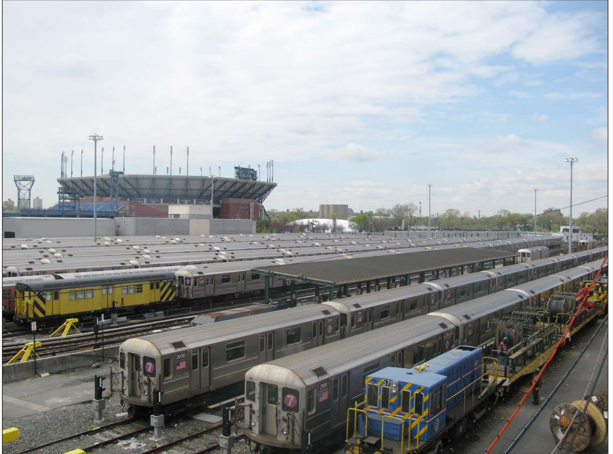
View from Passerelle Ramp to project site 25
