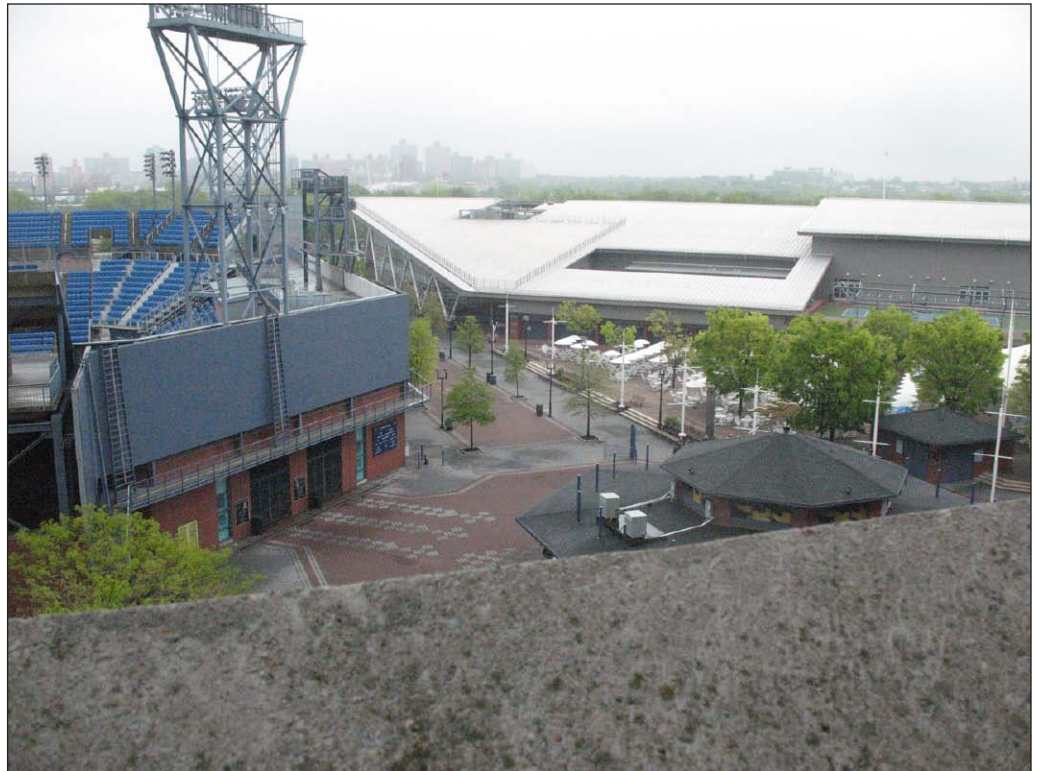
View from Arthur Ashe Stadium, facing east 1
