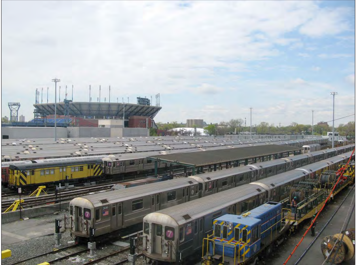
View from Passerelle Ramp to project site 25
