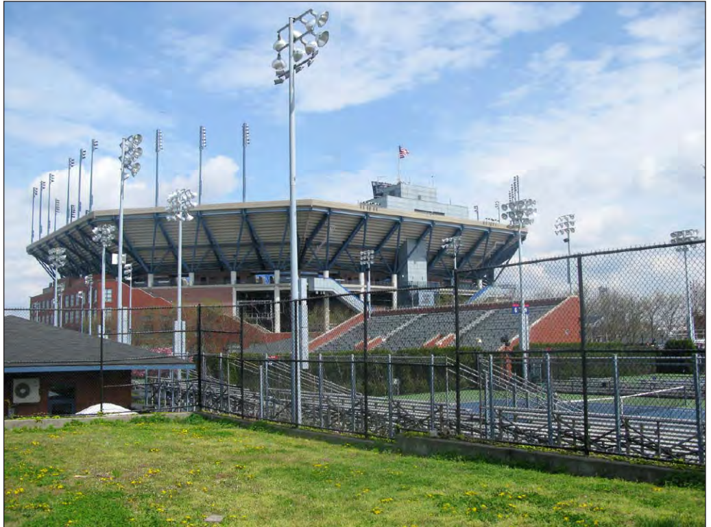
Southwest corner of National Tennis Center 7
